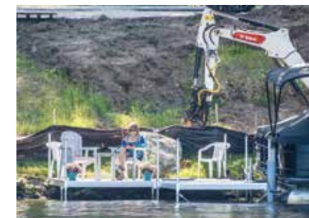
Joann at her dock during construction.
