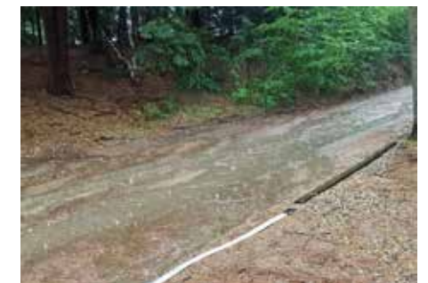
Pre remediation muddy stormwater runs down road towards streams during deluge.
